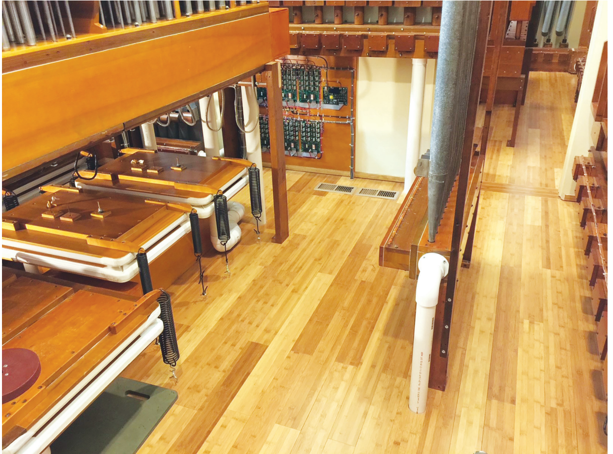
The Solo chamber: notice the wind conductors going through the floor (Photo courtesy of Ed and Patti Zollman)
